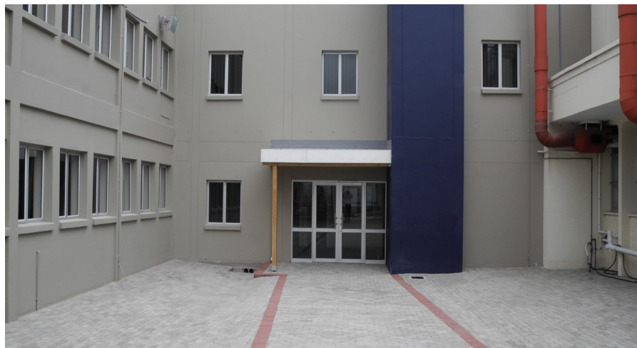
Entrance to InnoVenton's new Administration Building on Gomery Avenue
